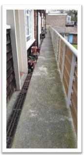
**The solution:** A programme of repairs was to be undertaken for both the staircases and balconies. Concrete repairs were identified and completed. A migratory corrosion inhibitor (MCI) was applied to the repair areas and to all other exposed concrete surfaces. Upon completion of the repairs, the staircases and balcony soffits and facias were thoroughly
